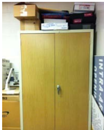
Unanchored Locker, [REDACTED] P&DC
