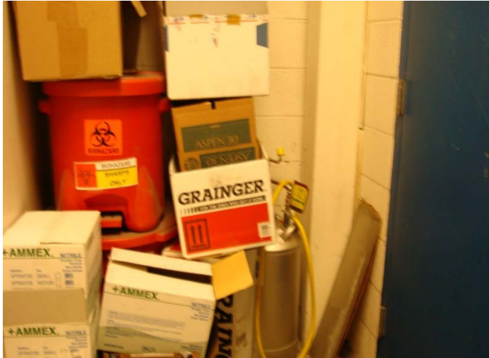
Figure 2. Blocked Eyewash Unit, [REDACTED] P&DC
